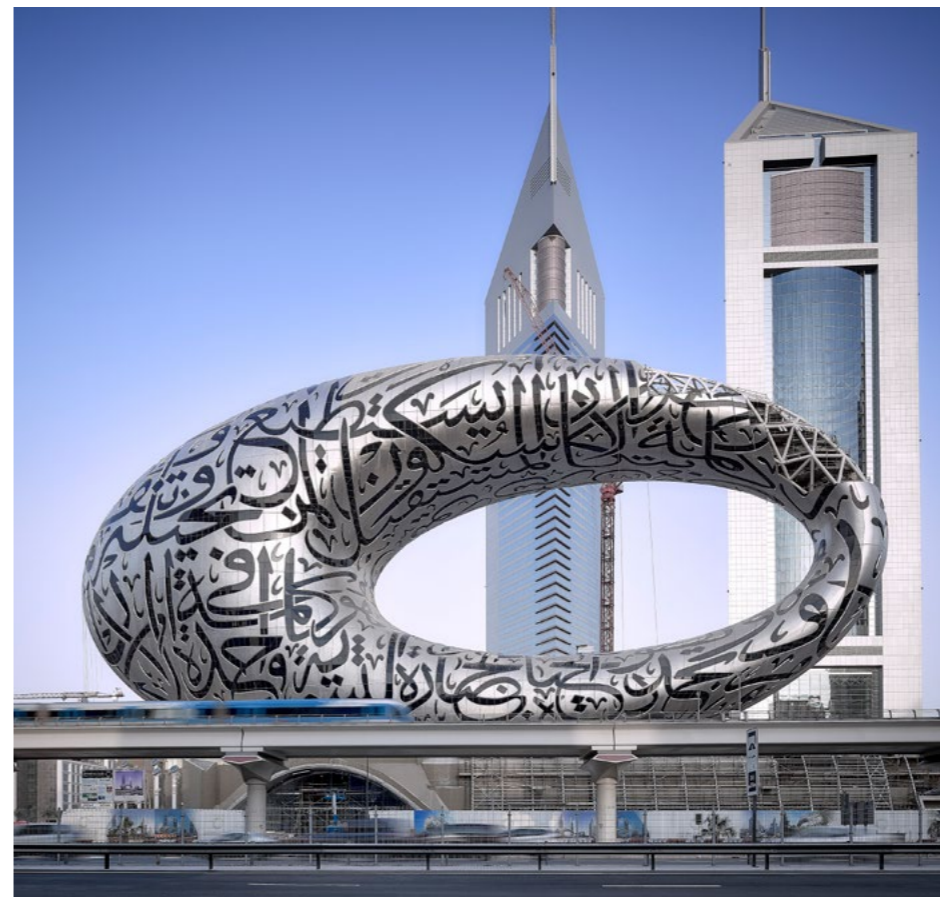
Buro Happold's Museum of the Future project. Photo: Phil Hanforth.
