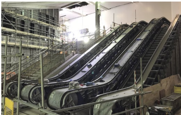
Escalators on the Crossrail project.
