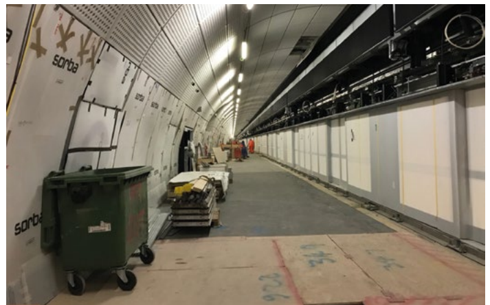
Station work on Crossrail.
