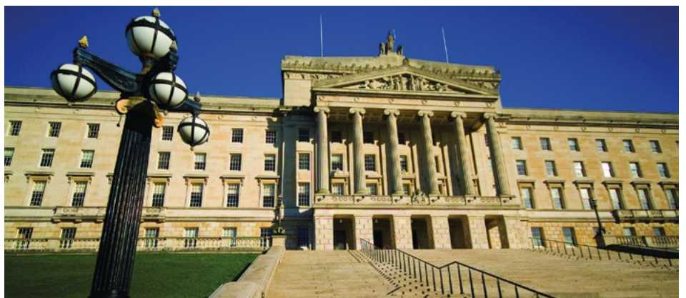
Stormont, home of the Northern Ireland assembly.
