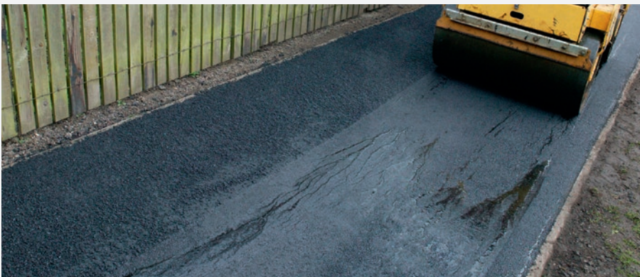
The footway Retread process in action in Peterborough
