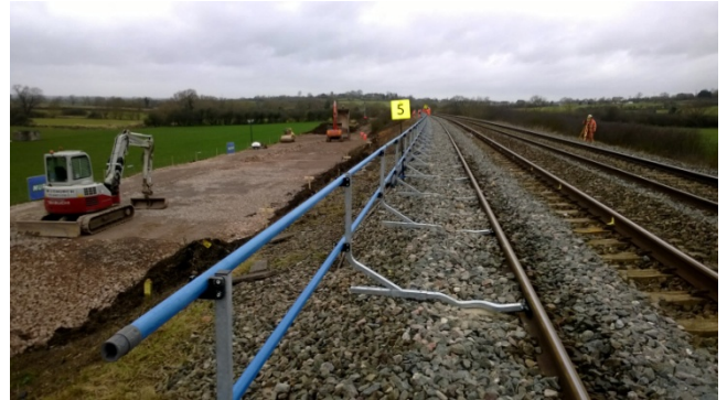
Section of track on Ladbroke Lane
