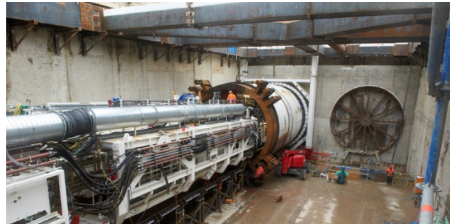
Crossrail Thames Tunnel C310 project
